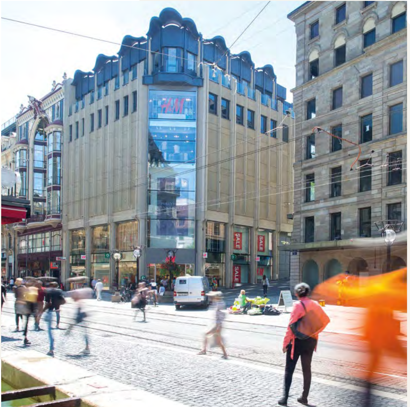
On the right side 40 Rue du Marché - a building currently under refurbishment.
