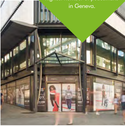
The impressive Snipes frontage before opening in Summer 2018
